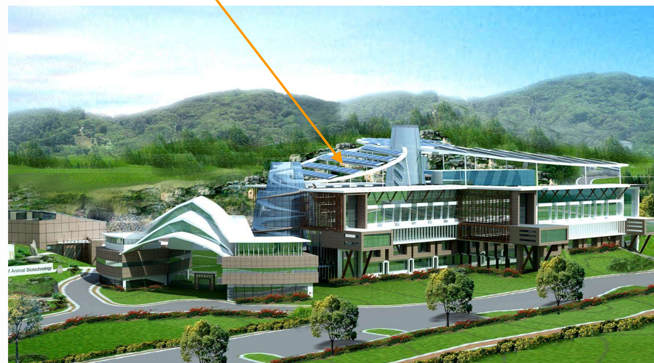
Fig 2 – Detail roof 3d over the courtyard with solar panels.
