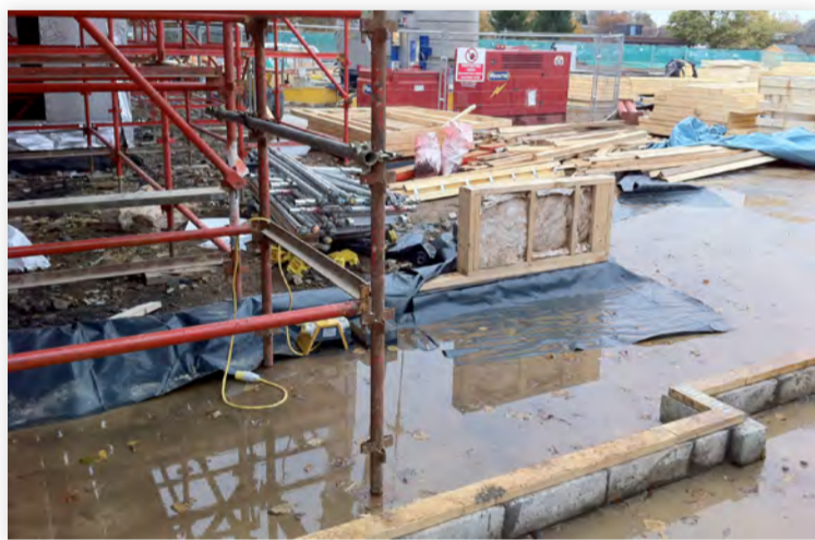
Wall plinth Construction
