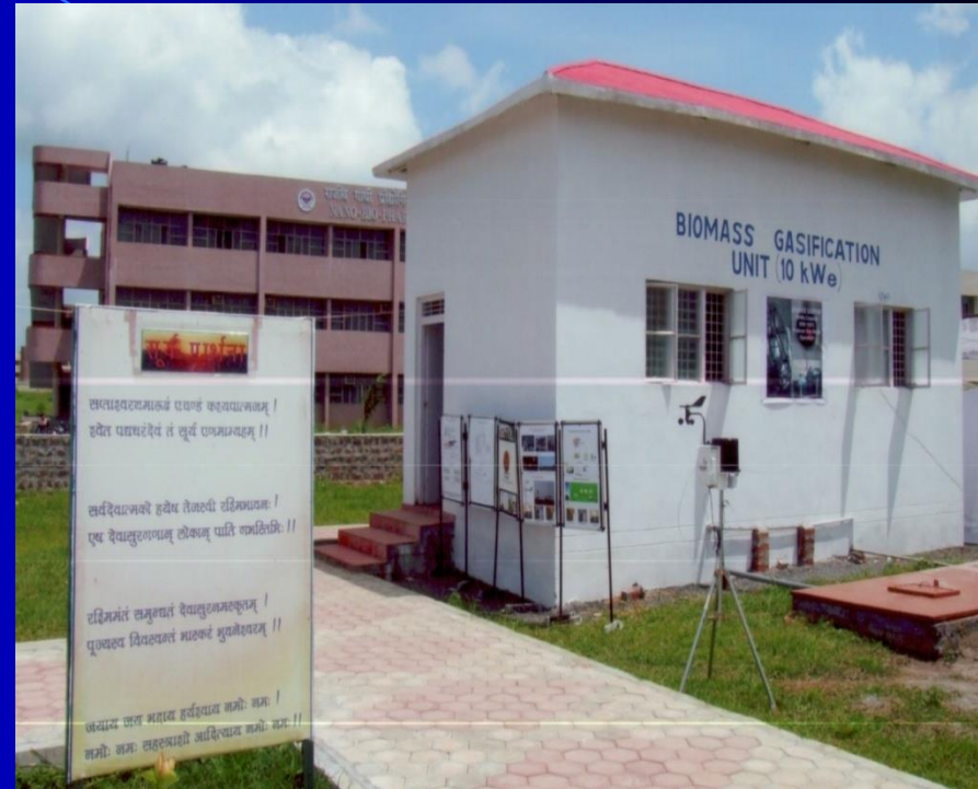
BIOMASS Gasification Unit
