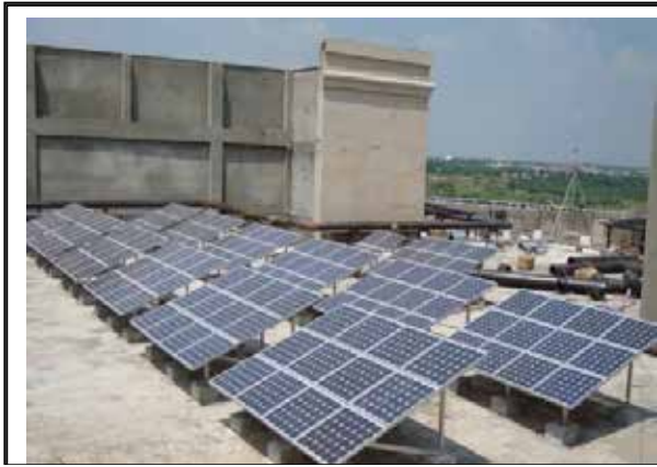
12 KWP SYSTEM INSTALLED AT DLF PROMANADE MALL - NEW DELHI
