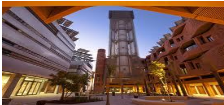
A ventilation tower using natural airflow World's First Zero Carbon City
