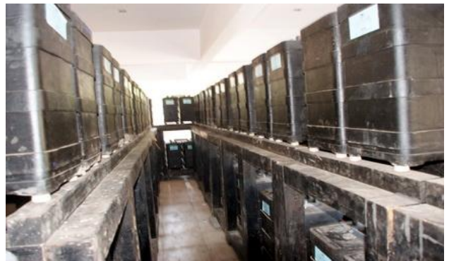
134.4 KWP SYSTEM INSTALLED AT R&B SURAT, GUJARAT
